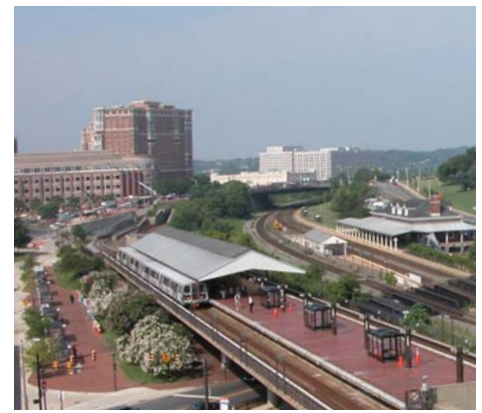
WMATA, King Street Station Improvements
